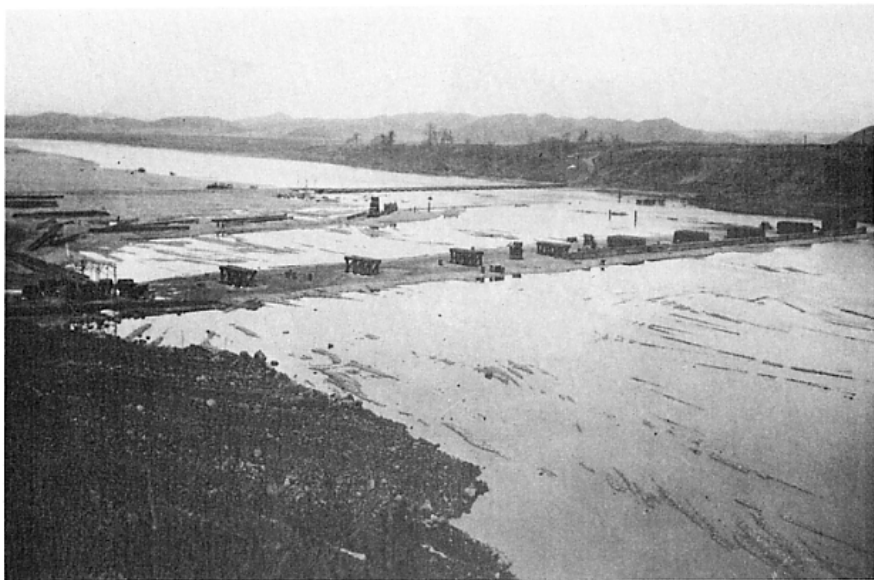
Figure 26. Teal site on 26 November 1952 showing completed piers at south end of bridge, left, and others still under shelters. I-beam girders and the Imjin River flowing north of the causeway are visible at right.
