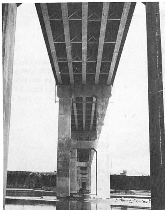
Figure 61. View looking east at the completed piers and superstructure of Libby bridge.
