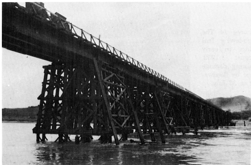
Figure 16. A survivor: the high-level Whitefront timber-pile bridge in September 1952 with damage largely limited to the fender piles.
