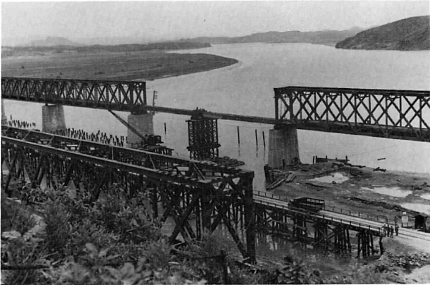
Figure 11. Construction under way to reopen the more southerly railroad bridge at the Freedom Gate site. The low-level pile bridge is visible at the right of this 9 July 1952 photo.
