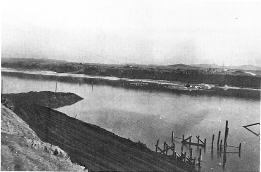
Figure 38. The Imjin River at the X-Ray site, showing early progress on the construction causeway and test piles driven in November 1952 to determine the depth of bedrock.
