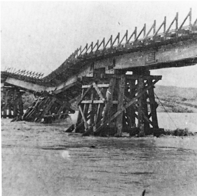
Figure 12. The high-level Teal bridge collapsing under the pressure of floodwater on 30 July 1952.
