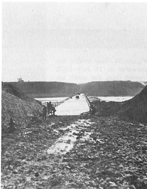
Figure 32. Teal bridge from the north shore on 16 January 1953 when almost completed. This view shows the removable guardrail.
