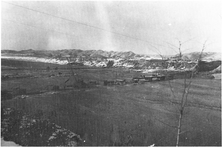
Figure 30. Girders in place on piers 8 through 11 allowing the passage of water below these spans and the construction of a causeway to pier 11 from the north bank.
