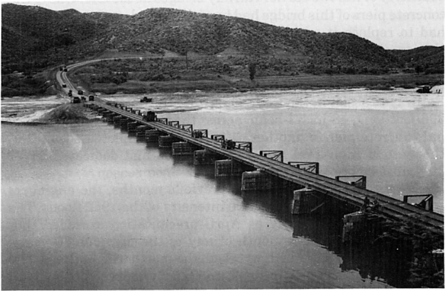
Figure 17. Spoonbill bridge on 20 June 1953.
