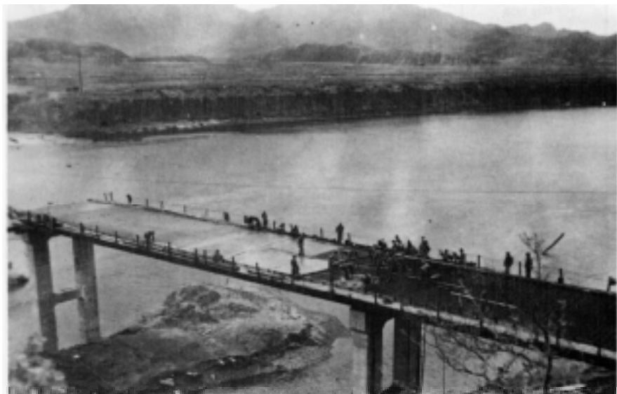
Figure 75. Troops laying the concrete deck. Two steel mats reinforced the concrete to provide an "antiartillery" safety factor beyond the necessary load-carrying strength. The concrete placing was monolithic and continuous.
