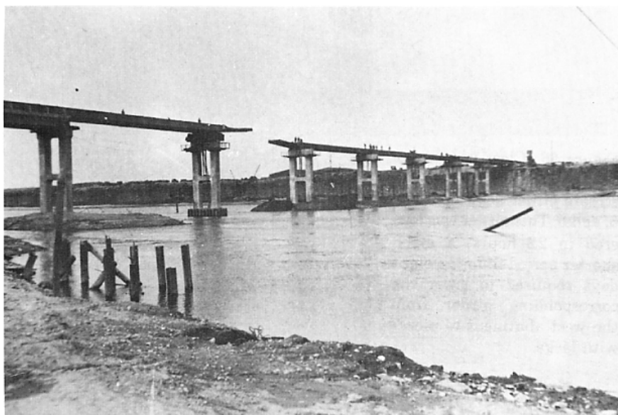
Figure 54. Launching the span across piers 7, 6, and 5. Launching noses extend both east and west into the gap between piers 5 and 6.
